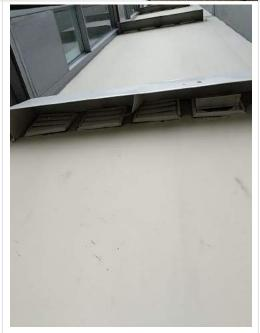
Vents dirty, cracked and in need of replacement. If left as is, birds can get into louvers and makes nests, which will block off the vent.
